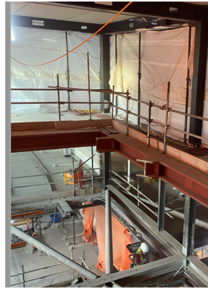
The installation of the steelwork at levels 6 and 7
